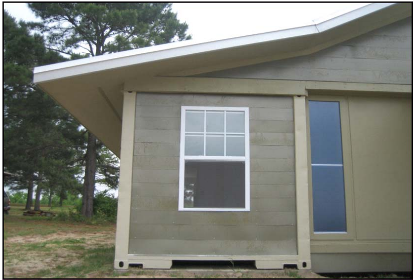
This Rural Studio house for families, developed by AIDS Alabama, Auburn University, and AIDS Outreach of East Alabama, uses railroad cars for bedrooms.
